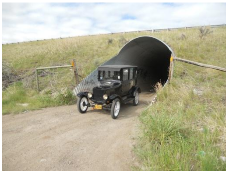
Culvert driving under free way
